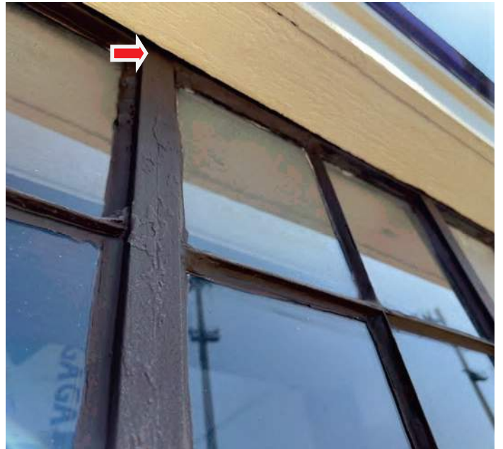
Photo 16: View of brown paint on wood - upper level window framing.
