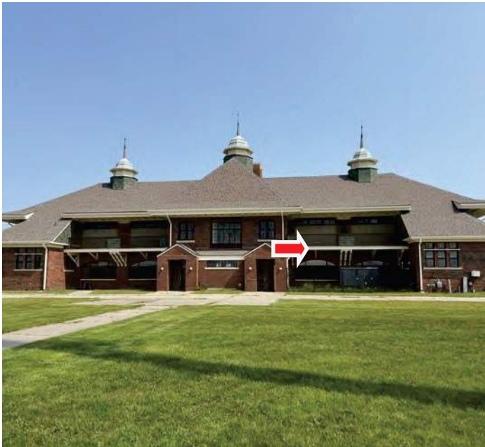
Photo 11: View of light cream paint on wood fascia boards/trim.
