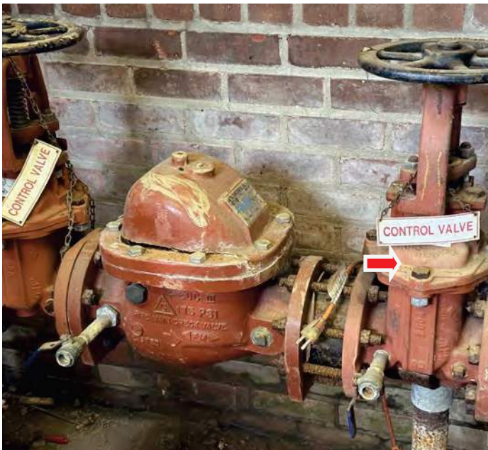
Photo 3: View of assumed ACM pipe flange gaskets.
