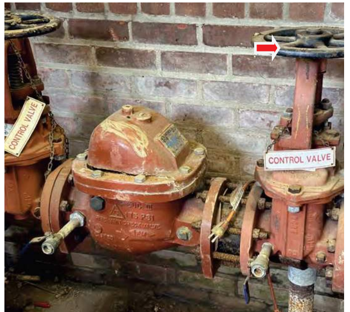
Photo 4: View of assumed ACM pipe valve packings.
