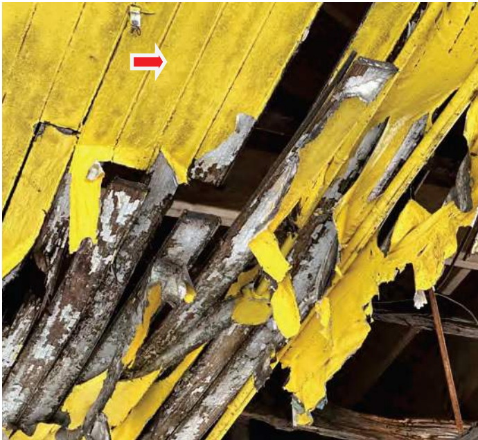
Photo 22: View of light yellow paint on wallboard walls.
