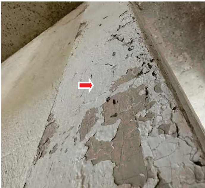
Photo 26: View of white paint on wood-door framing at upper level.
