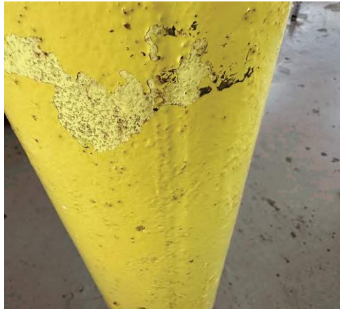
Photo 31: View of yellow paint on metal-support columns.
